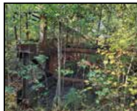
Large Bridge Transport Steel Structure
