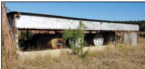
Steel Tank Storage Structure
